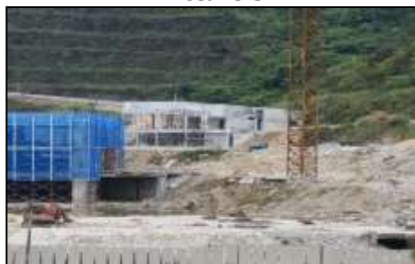
- Construction Work Underway in Genting Highlands Area
