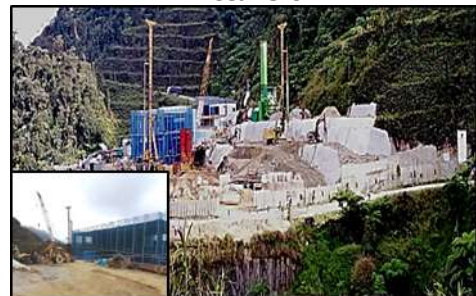
- Construction Work Underway in Genting Highlands Area
