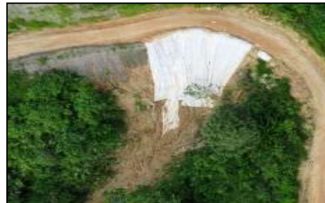
Temporary Soil Stabilization Not Done in Exposed Areas Transmission Line Project Causes Soil Erosion and Landslides
