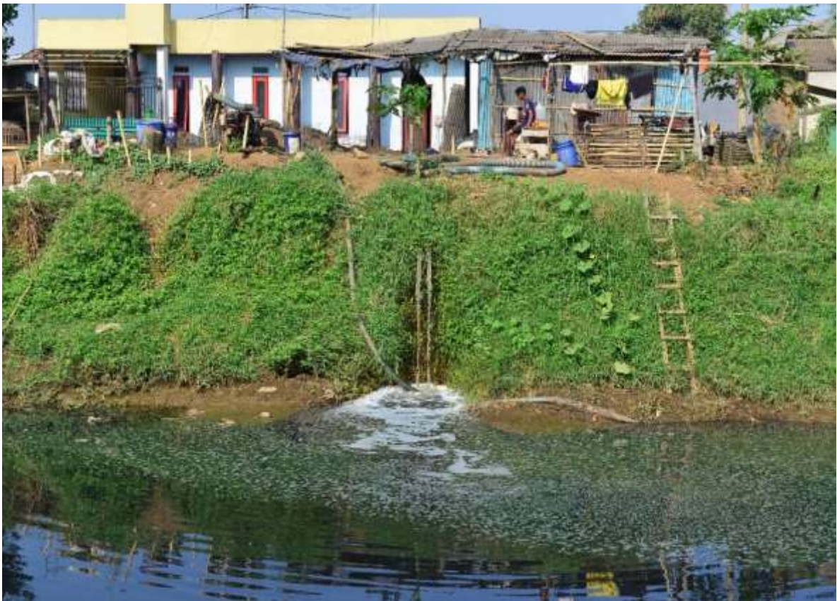
Figure 4. Domestic Wastewater Pollution on Citarum River
